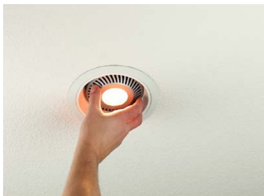
Photo 6 Indoor lightning (source, BanksPhotos/Getty Images)
