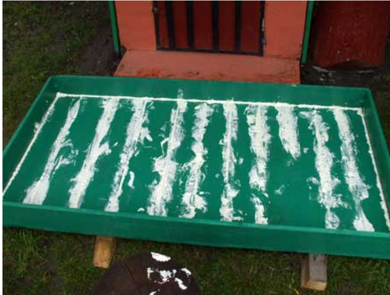
Photo 9 The isolation of the wood box with polyurethane foam (source, http://www.douamaini.ro/ )
