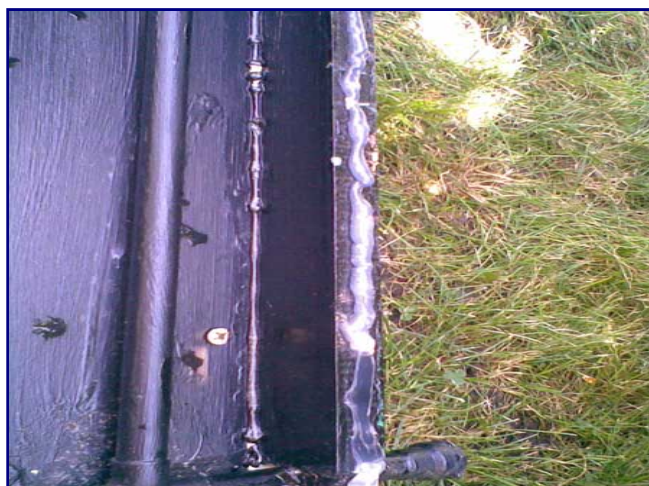
Photo 14 Sylicon sealing (source, http://www.douamaini.ro/ )
